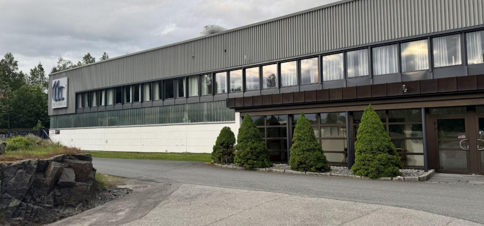
TTC Norge's facility in Slitu, Norway, where SCM Frigo installed two SMART Heat Pumps. Photo credit: SCM Frigo
